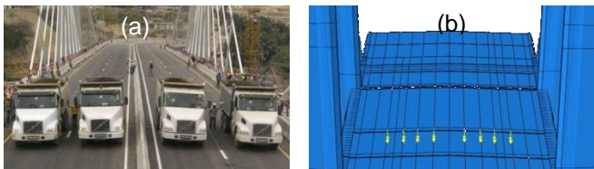
Fig. 7 – Static loading tests: on-site (a) and in the numerical model (b).
