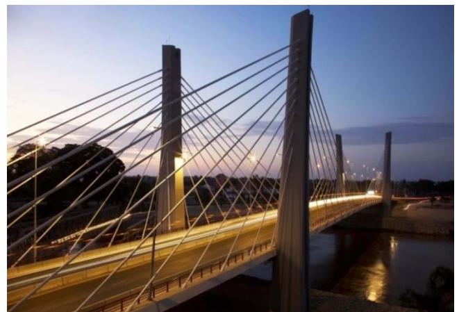
Fig. 1 – View of the “4 de Abril” bridge.
